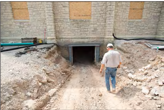
A temporary access point and ramp to the below grade expansion was created at the east side of the church.
