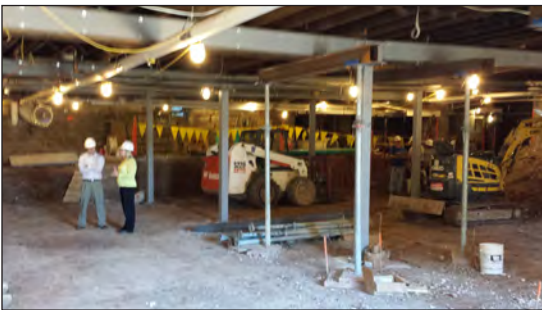
Expanding underneath a 100+ year old structure required a tedious shoring and excavation sequencing plan.
