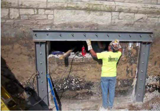
A temporary access point and ramp to the below grade expansion was created at the east side of the church.
