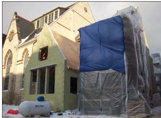
Expanding underneath a 100+ year old structure required a tedious shoring and excavation sequencing plan.
