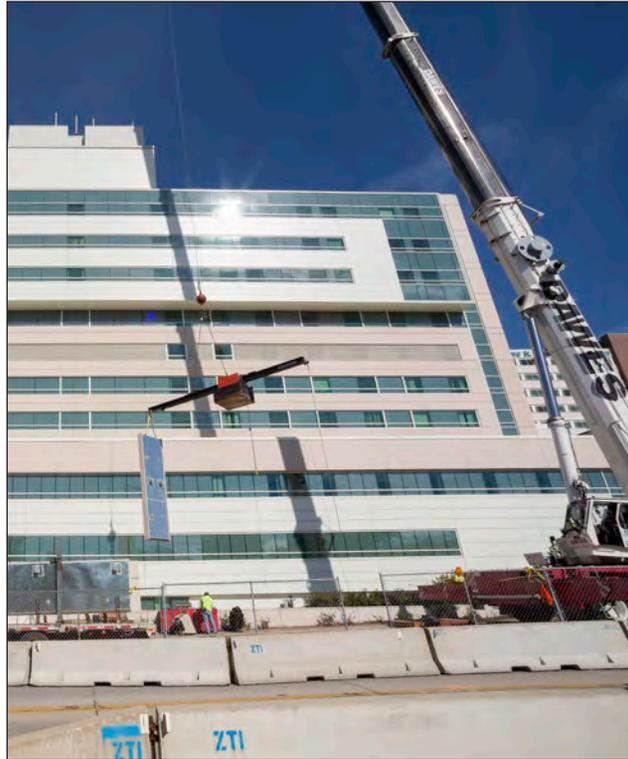
Use of the “Flying Jib” allowed panels to be installed beneath upper floor projections. This panel is on its way to being installed “in the blind” on the opposite side of the building.
